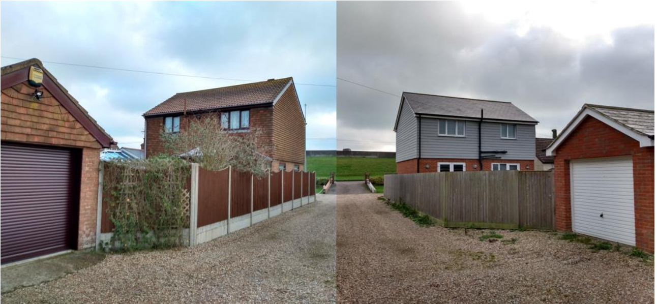
Photo 4: Rear of 1 and 2 Willop Close
